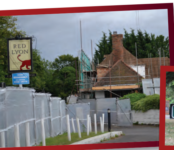
Red Lyon, under refurbishment
